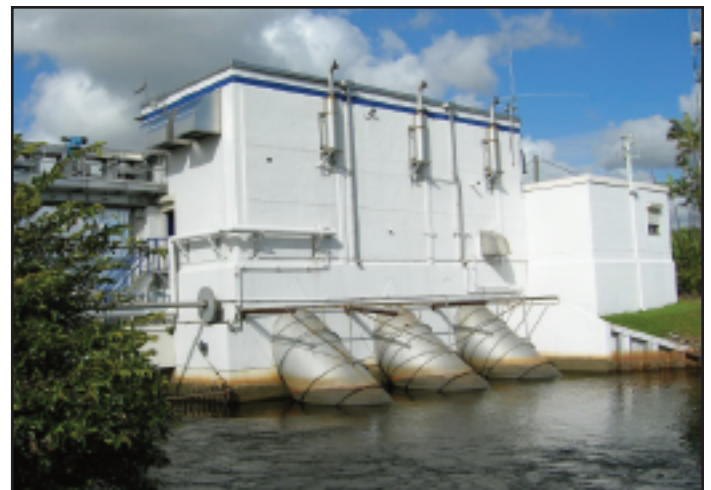
Figure 7 - S-13 Pump station located on C-11 canal in Davie, FL. It has a rated capacity of 540 cubic feet per second, equivalent to approximately 14.5 million gallons per hour (Credit: SFWMD).
