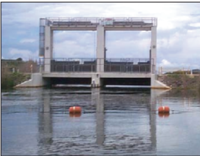
Figure 6 – Typical coastal flood/salinity control structure of the sluice gate type. (Credit: SFWMD)
